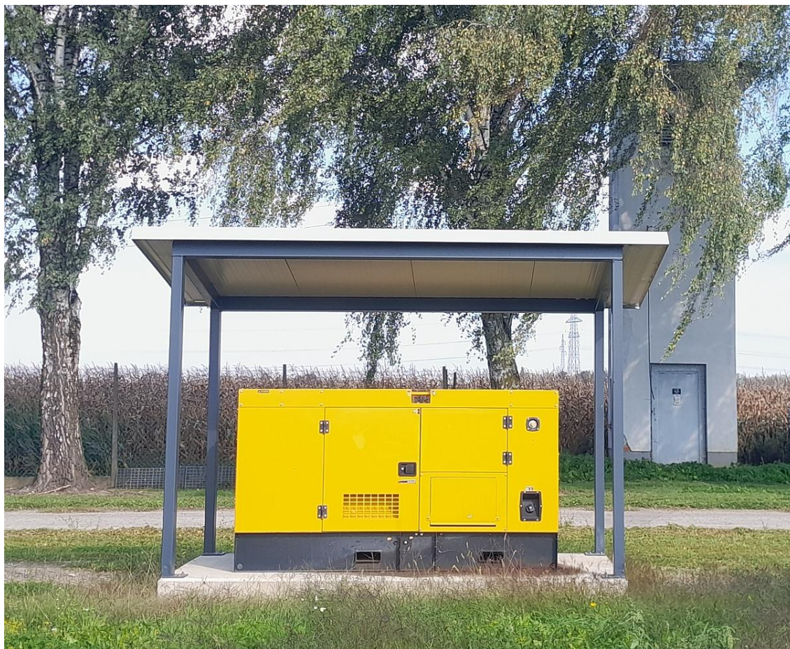
Diesel generator in transformers station
